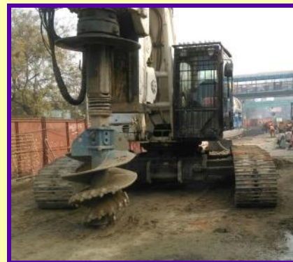
Foundation, Piling and Geotechnical
